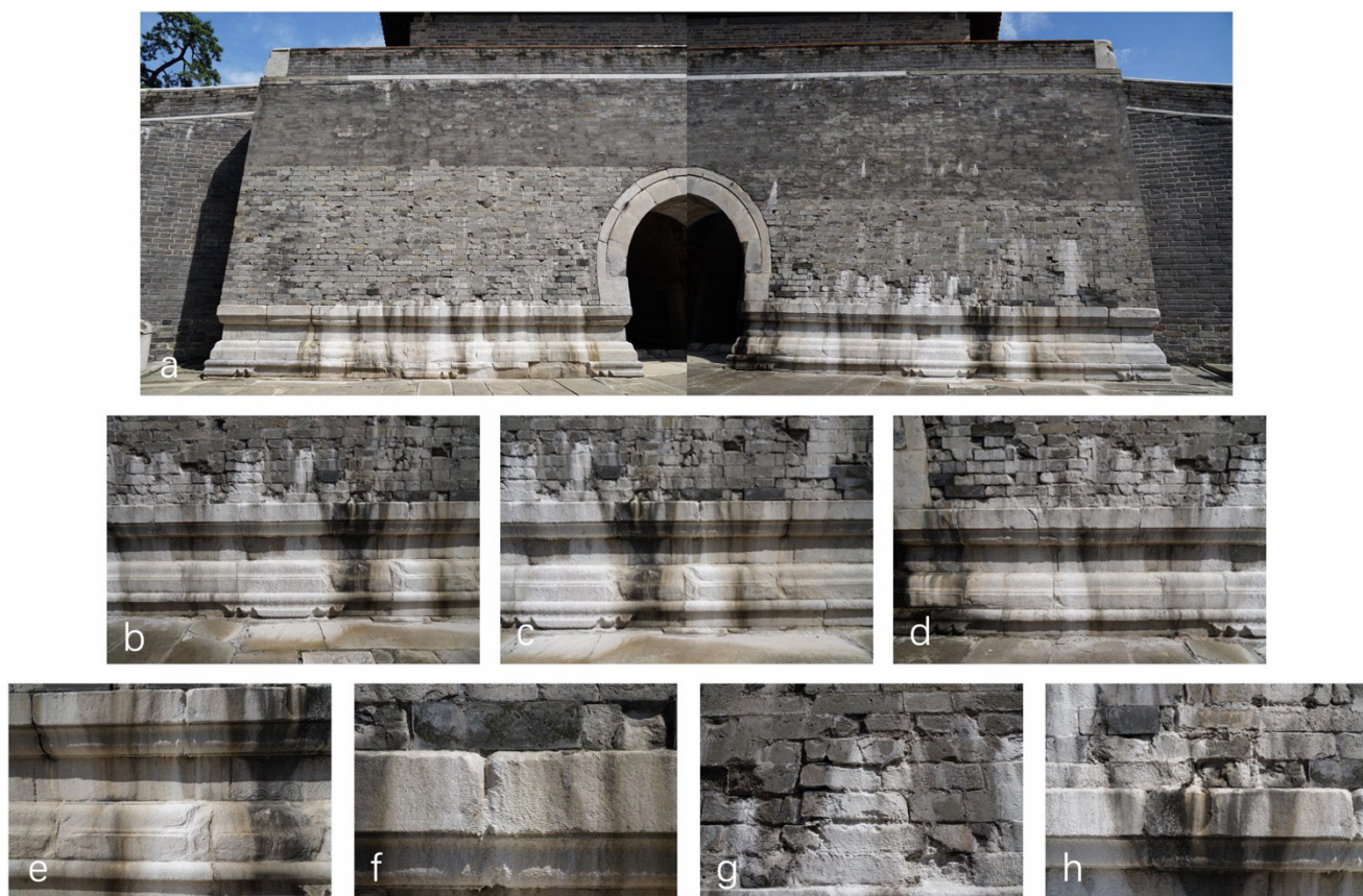
Fig. 9 Visible salt deposits and their spatial distribution on the Square City at the Ming Dynasty Kangling Tomb: (a) Overall view of the façade showing the affected areas; (b) Salt deposits and dark staining on the left-hand section of the Xumizuo and adjacent brickwork; (c) Salt deposits along the brick–stone interface and joints of the Xumizuo; (d) Distribution of salt deposits across the right-hand section of the Xumizuo and adjacent brickwork; (e) Close-up of dark staining and white deposits on the Xumizuo; (f) Close-up of white deposits along a vertical joint between stone blocks; (g) Close-up of white deposits on the brickwork and mortar joints; (h) Close-up of white deposits and dark streaks at the brick–stone interface. (Source: Photographs by the author.)
