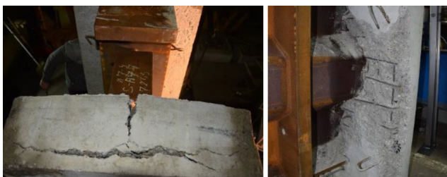
Fig. 3 Failure modes: slab opening and concrete crushing
