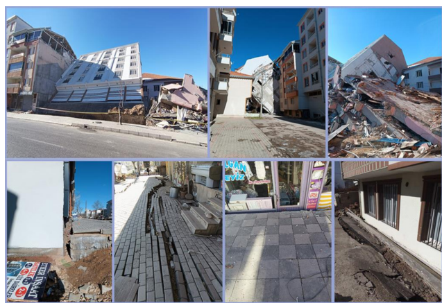
Fig. 2 Examples of structural damage caused by settlement and loss of bearing capacity due to seismic liquefaction in Gölbaşı, Türkiye [2, 5, 6]
