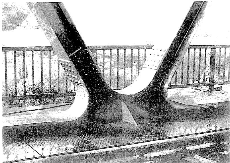
Fig. 9. One of the joints of the railway bridge at Bánréve
