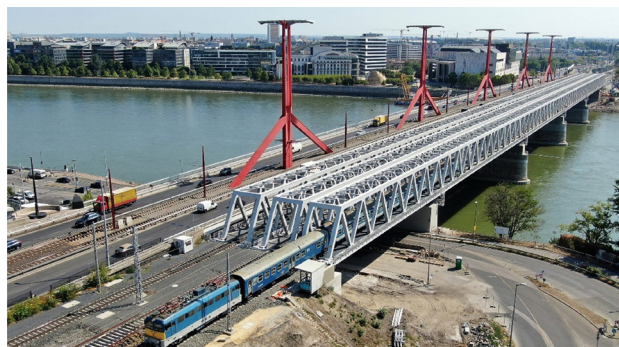
Fig. 1 Aerial view of Southern Railway Danube bridge
