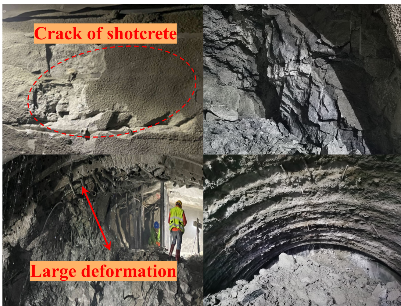
Fig. 1 The field rock layer joints and engineering disaster
