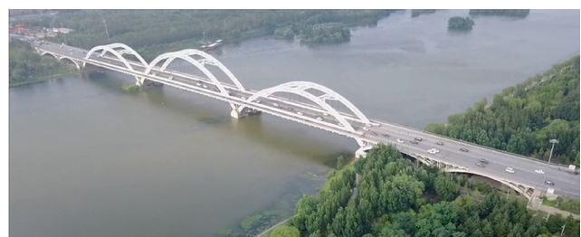
Fig. 1 Chang-Qing Hun River bridge
