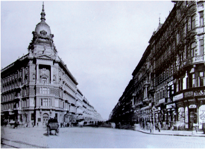
Fig. 6 The building in 1896 (BTM Photo archive, No. 2198033.)
