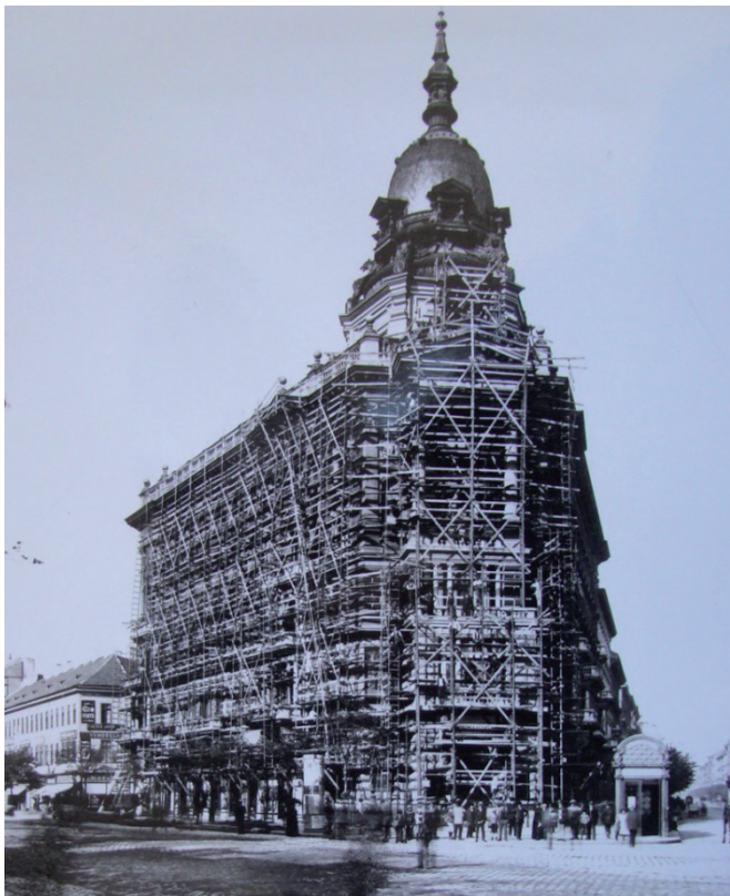
Fig. 7 Reconstruction works in 1900 (BTM Photo archive, No. 85.1739.)
