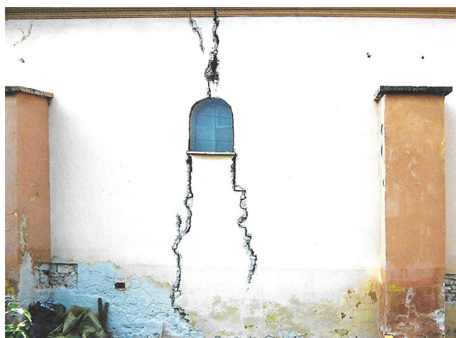
Fig. 4 The cracks on the southern facade of the Saint Michael Church before the restoration (Source: Armuth et al., 2016)
