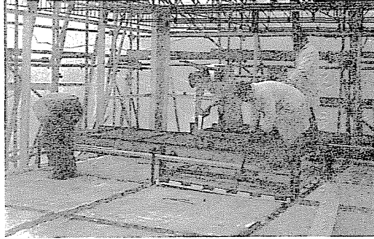
Photo 23. Location of reinforced top-of-cell elements. Folding out reinforcing stripes.
